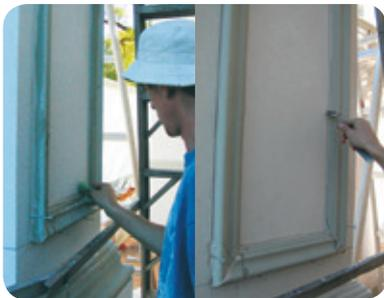
**6.3** Using the water and the brush clean away any excess remaining. It is important that when cleaning, a flush corner with no surface glue is the result for the best finish. Don not leave a groove between the moulding and the wall as this will show up when painted.
